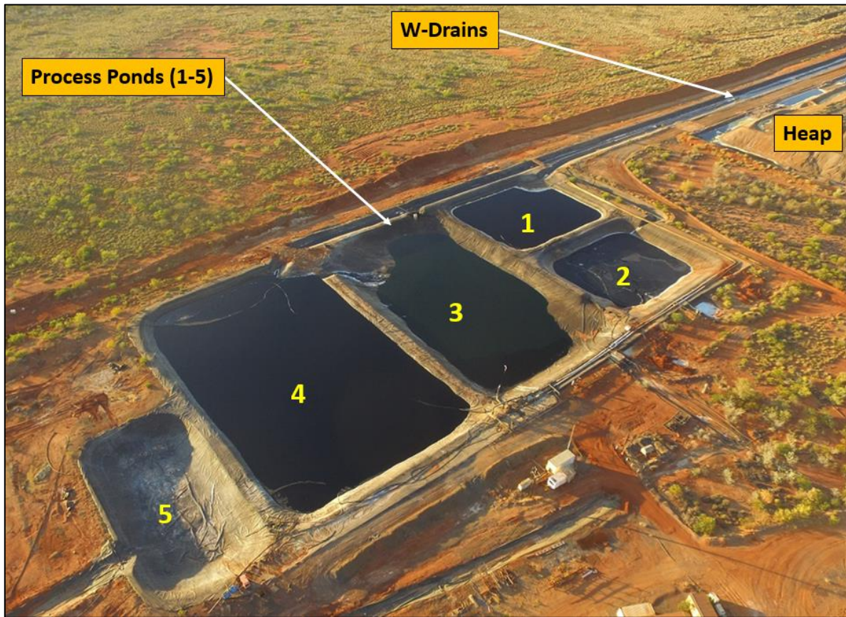
Figure 3: Process ponds 1 to 5 and W-drains now cleaned and certified
