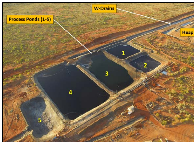
Figure 1: Process ponds 1 to 5 and W-drains cleaned and certified
