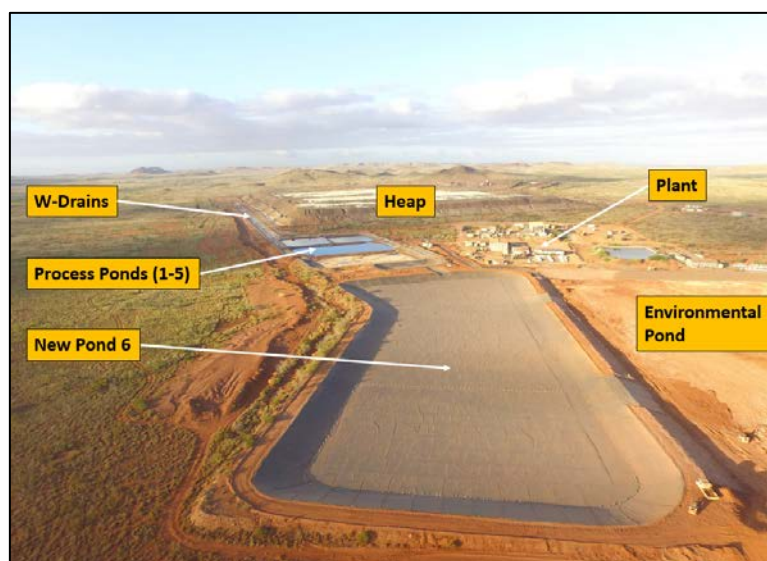
Figure 2: Pond 6 in relation to existing infrastructure
